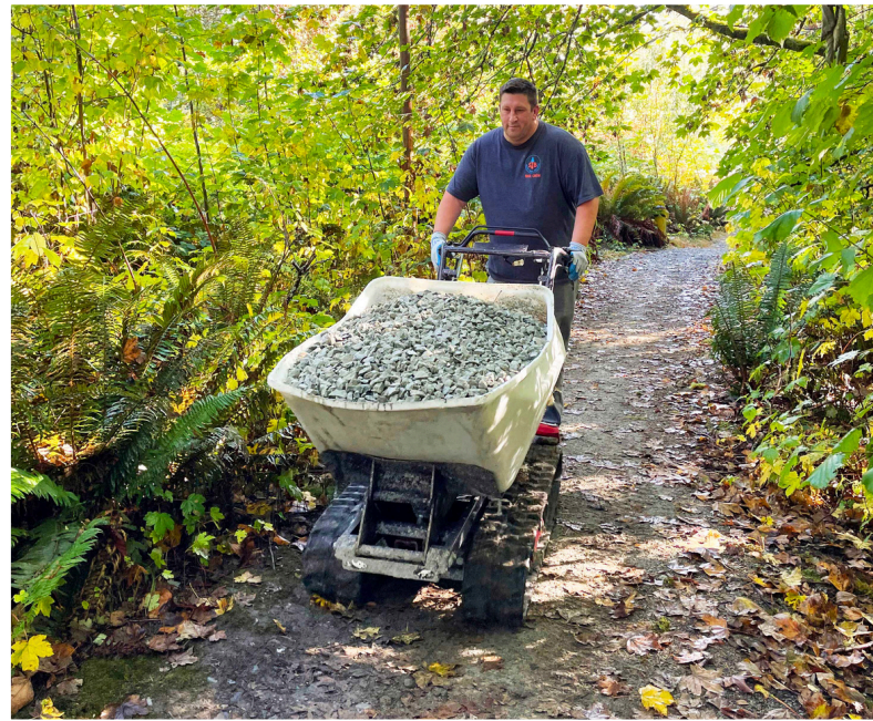
Pump House Trail, 2021-22
