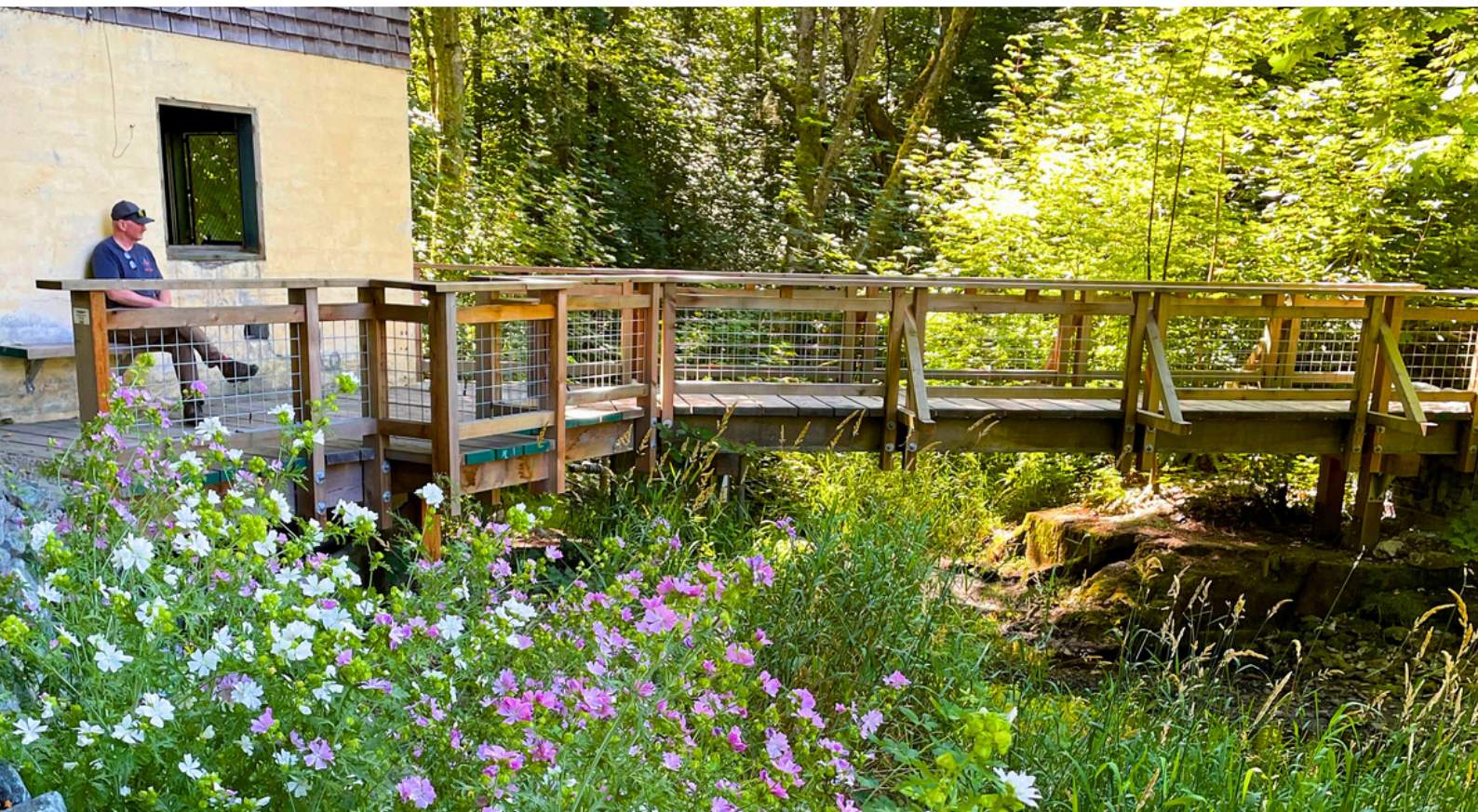
Pump House Bridge, 2022
